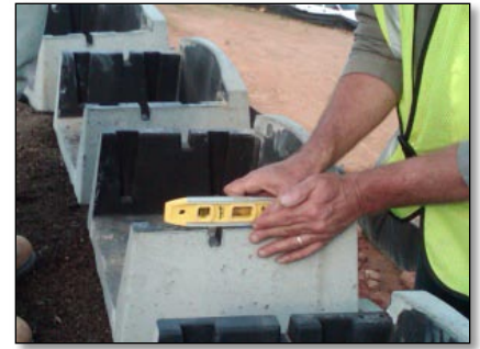
Checking Level Front to Back
