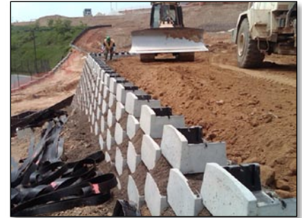
Installing a Lift
