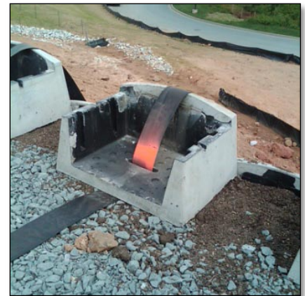
Correct Lower Strap and Backfill
