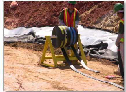
Spool Rack and Strapping
