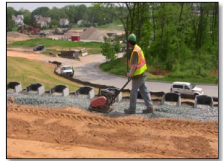
Vibratory Plate on Granular Zone
