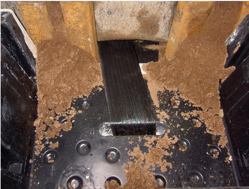
Figure B-4. Close view of the connection between ParaWeb and SmartSlope block.
